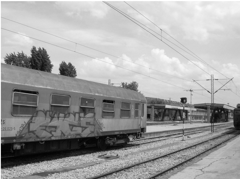
Fig. 9 – Railway station with 25 kV overhead line.
