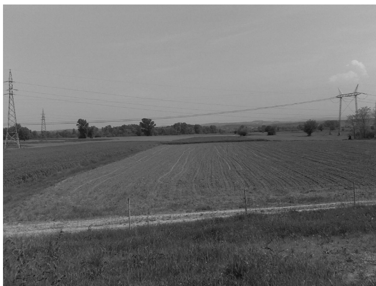
Fig. 8 – High voltage line sag due to heat.
